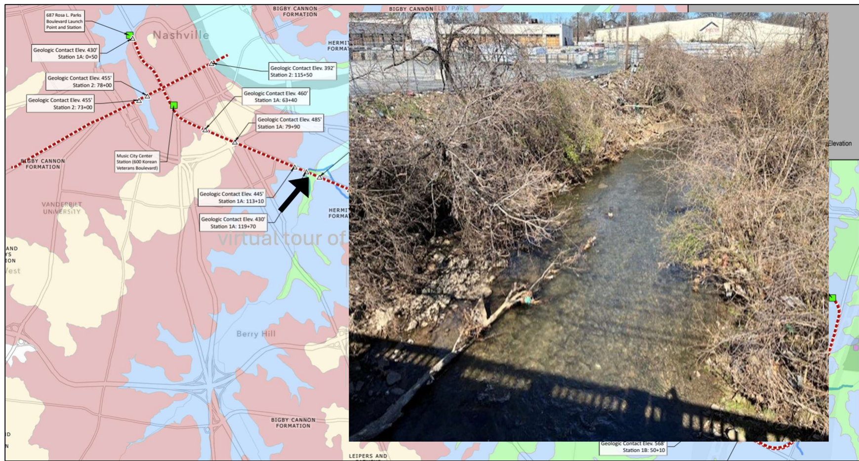
Figure 26. Crossing over Browns Creek which has cut its valley all the way down into the Carters Limestone (photo CG). Due to both well-developed karst in the Carters Limestone and saturated conditions beneath the water table, tunneling beneath Browns Creek will be challenging.
