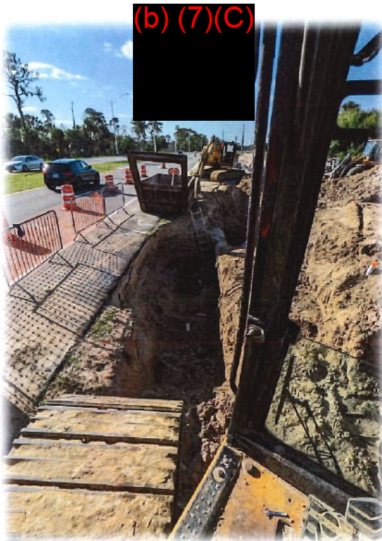
View from Excavator cab of the trench
