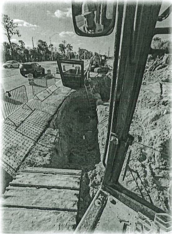
View from Excavator cab of the trench
