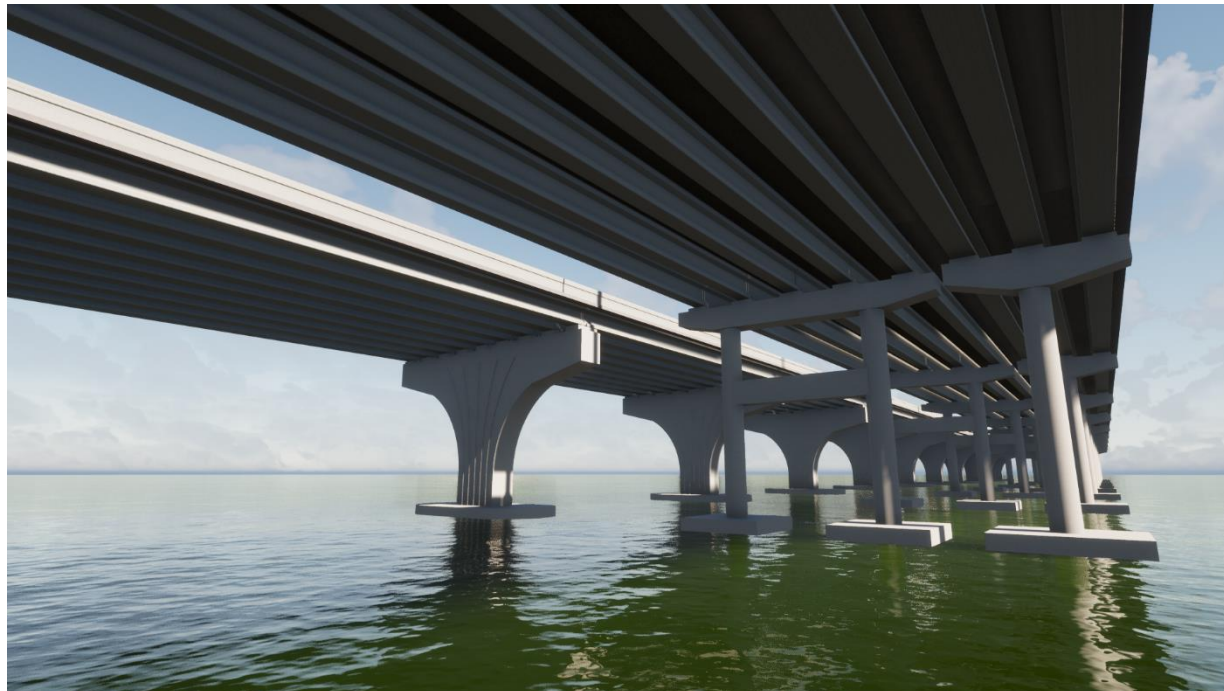
Pier Elevation View (Hammerhead Pier Option)
