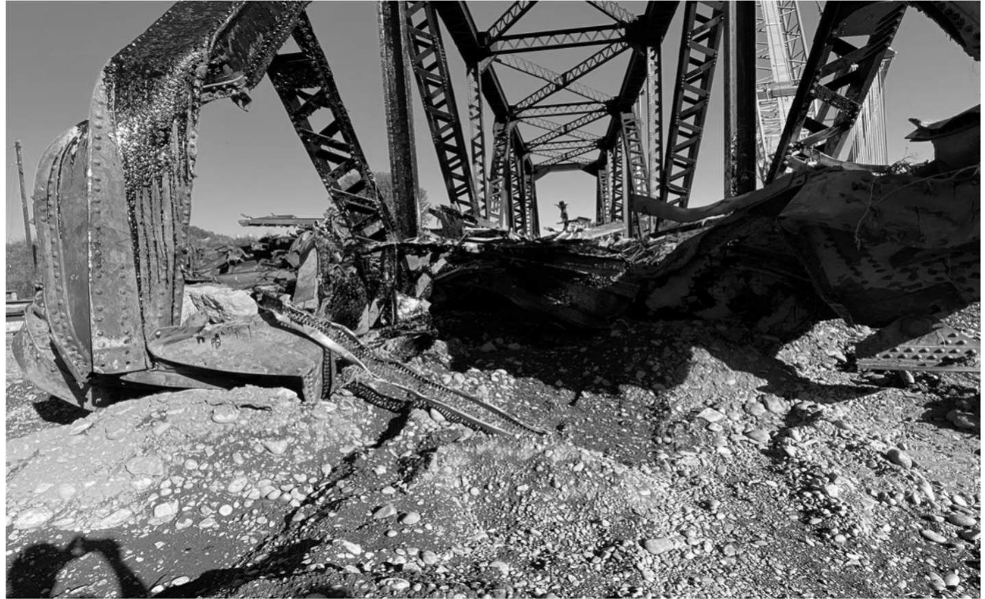
Car 38 (UTLX665072) and the damage that was caused to span 3 by the impact
